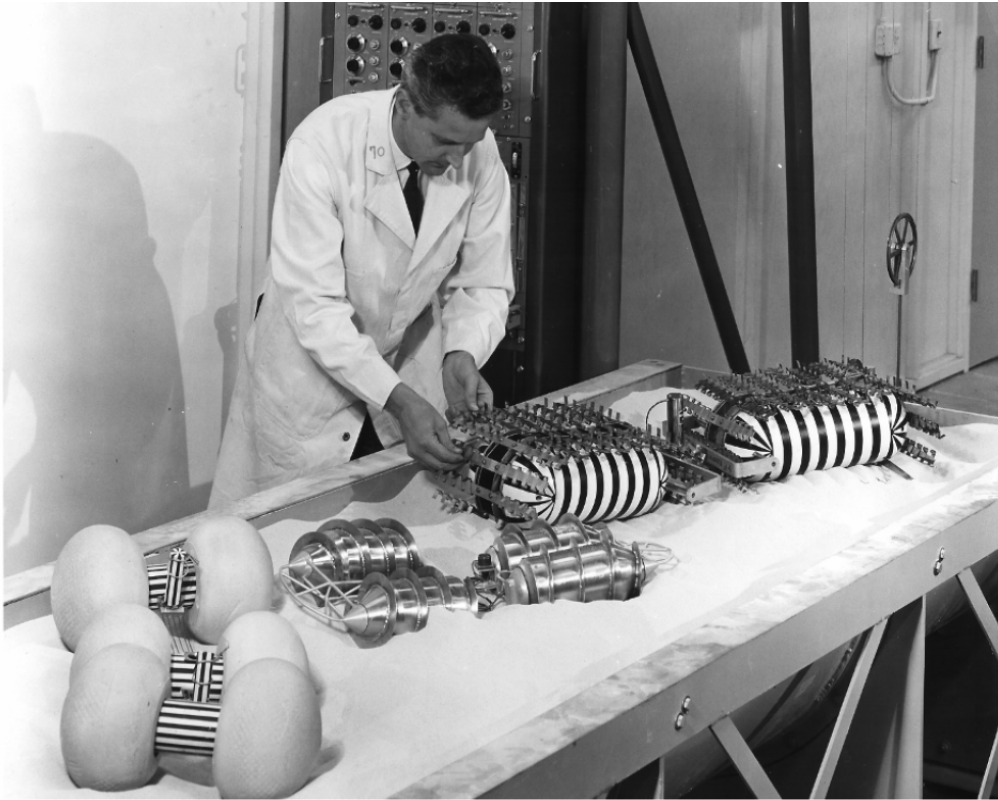
Figure 1. Three Types of Lunar Mobility Approaches Including Screws
